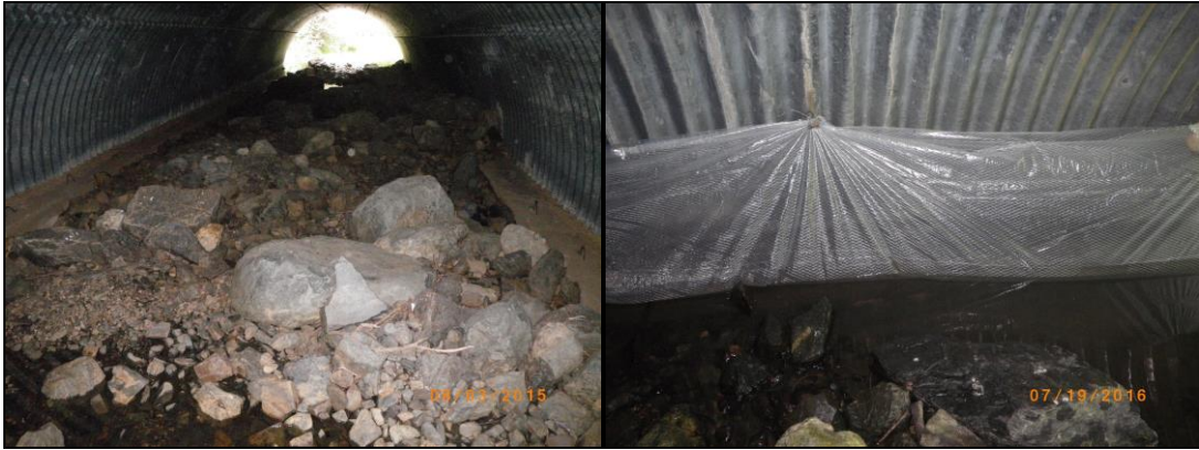
Figure 5. Resorted stream simulation material prohibiting passage through the Battle Creek Culvert (left) and plastic sheeting 'purse' passing stream flows during implementation.
