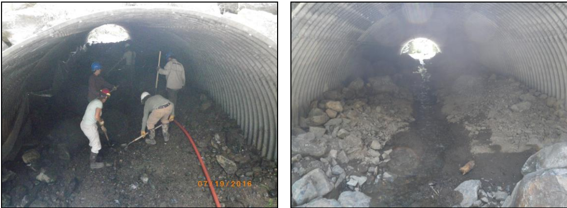
Figure 6. Youth crew excavating the low flow channel within the inset floodplain (left) and the finished inset floodplain and low flow channel.
