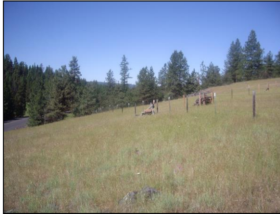
Figure 7. New fence constructed on a hillslope above Camas Creek and its floodplain.
